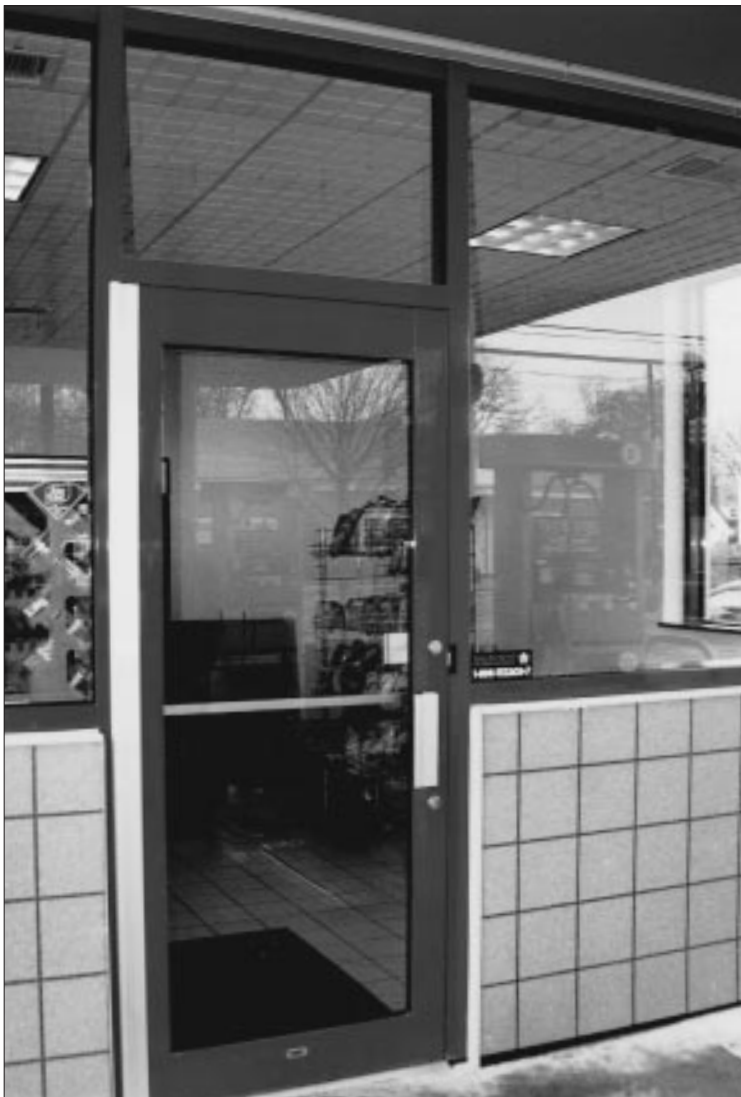
Bullet Resistant Door with Transom and Electric Release System
